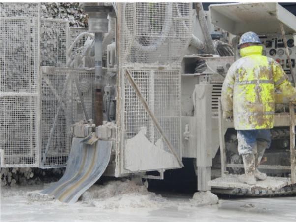
Both heat pumps are attached to an array of boreholes drilled in the Autumn of 2011 in the garden area adjacent to the swimming pool. Each of the 11 boreholes is drilled over 100m into the chalky bedrock formed over 90 million years ago in the Cretaceous Period. The water present in the chalk resulted in the drilling rig, operator and part of the garden being turned temporarily into a winter wonderland scene.
